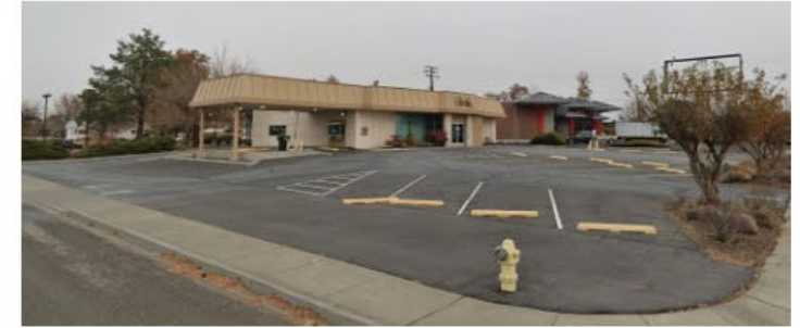
E VIEW FROM N 11TH AVE
