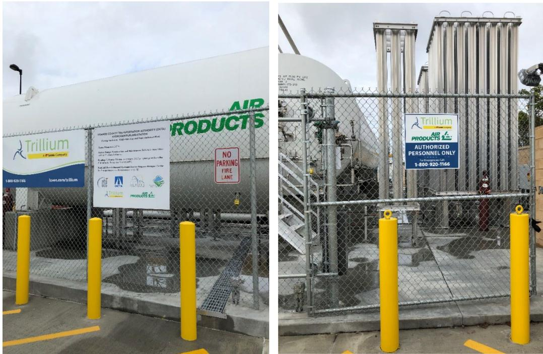
**Figure 39: Liquid hydrogen storage tank and vaporizers as part of Orange County’s hydrogen fuelling infrastructure.**
