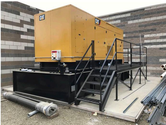
If BFT wishes to operate for more days during an emergency, the size of generator will stay the same, but the required quantity of fuel will scale linearly. The total amount of fuel required to be stored onsite will depend on the anticipated duration of the utility electrical outage and the amount of time required to get a fuel delivery of diesel fuel, as well as on environmental regulations and local policies.
