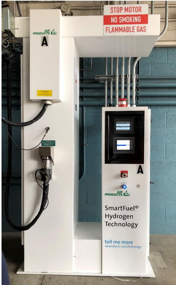
**Figure 40: Hydrogen fuelling dispenser, Orange County, California.**
