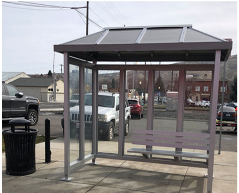
Figure 22: Two-tone Shelter at Stacy Ave. Transit Center
